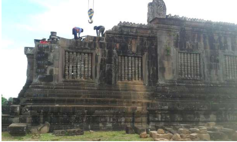
Beginning of the eastern porch restoration ( April )
